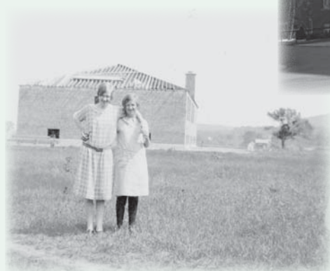
The picture above shows Henry Ellers under construction. At right is the building as it looks today.
