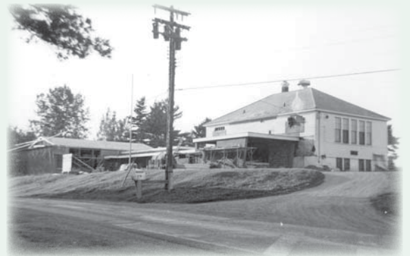
The old, wooden 1925 Pine Grove School (right) is shown during the construction of a new brick addition (left) in the 1950s.
